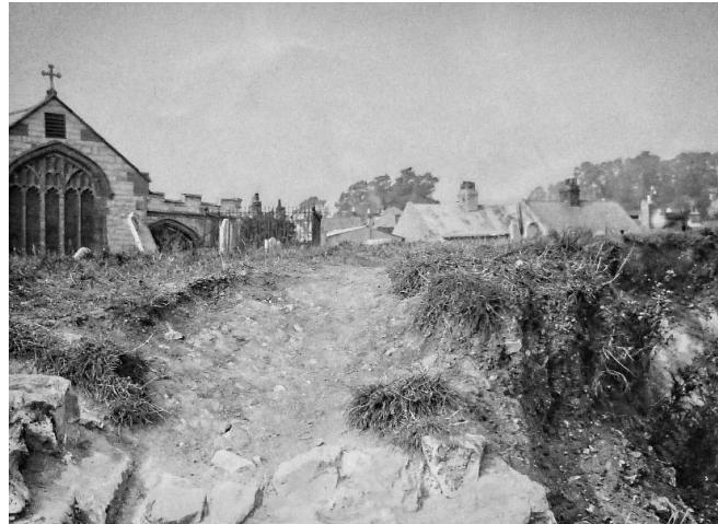
Continuing erosion of the churchyard shown in this 1909 photo
